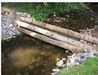
Fig. 2 Example of a leaky debris dam taken from [3]
