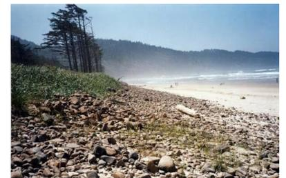
**Figure 3:** Dynamic revetment (cobble berm) completed in Oregon [4].
